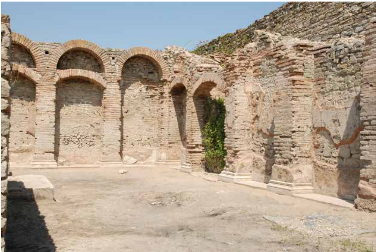
Fig. 73d. Building with Arches (Library), view of the arches on the north wall of the large hall
