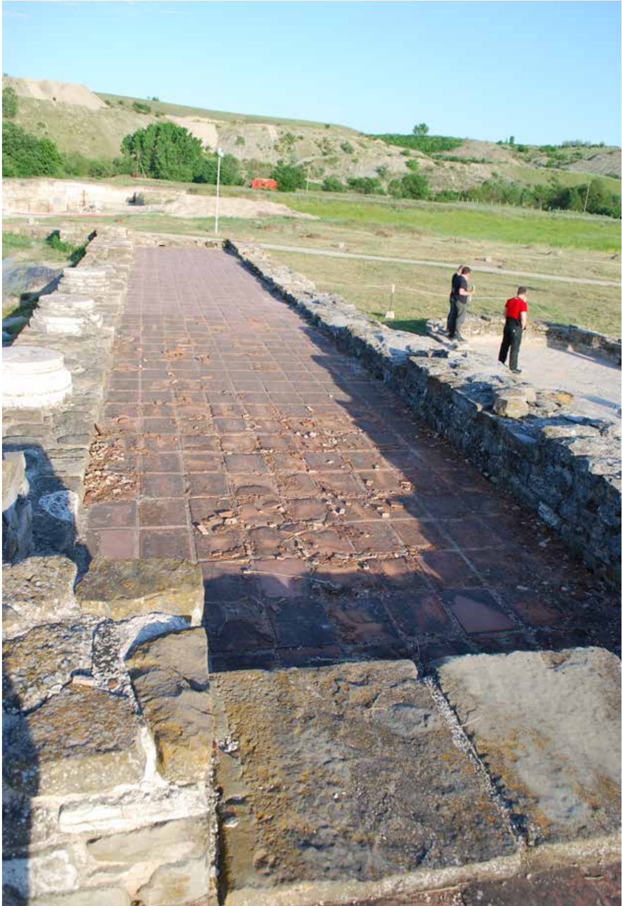
Fig. 54. Human hazards: an example of degradation of ancient features due to lack of maintenance
