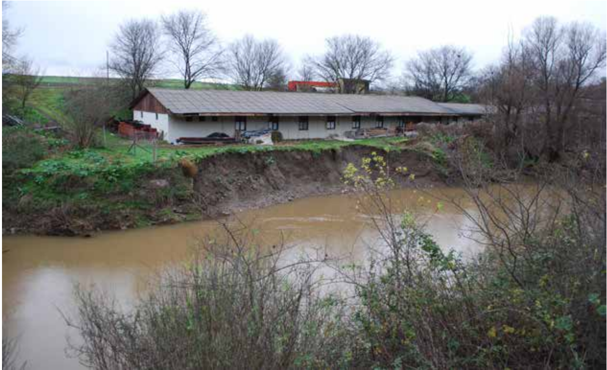
Fig. 38-39. Risk from flooding: collapse of the bank of Crna River adjacent to Depot 5, 2014
