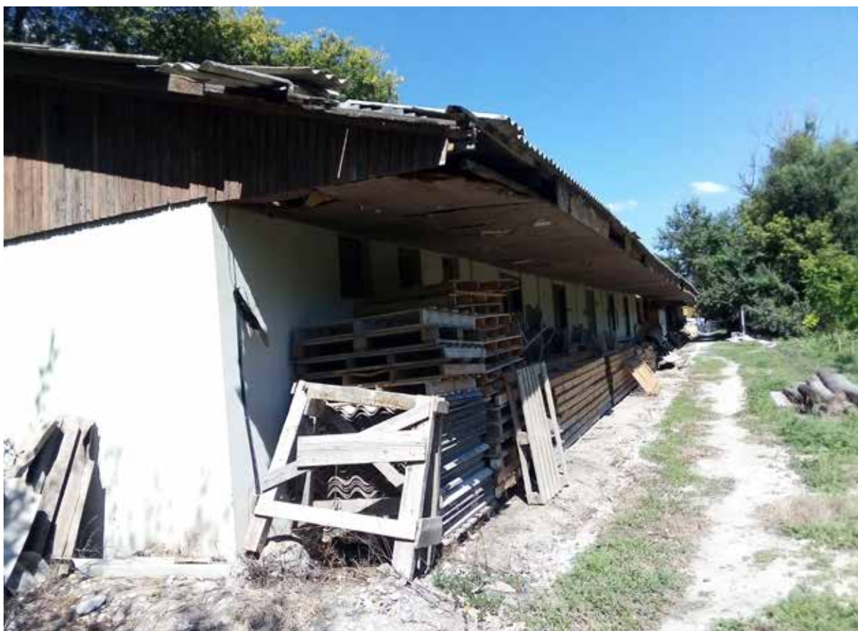
Figs. 102a-d. Storage facilities: depot 5 used for storage of study material and tools
