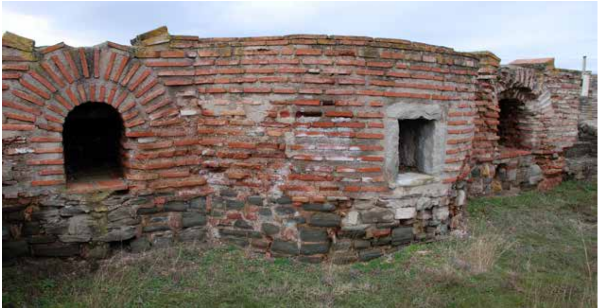
Fig. 87d. Large Bath, the praefurnium
