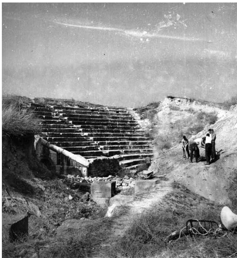
Fig. 12. Excavations of the Theatre in the 1930s
