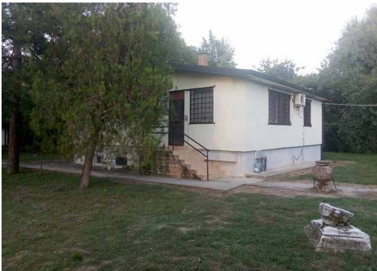
Fig. 101a. Main office: depot 2 is in the basement of the cabin
