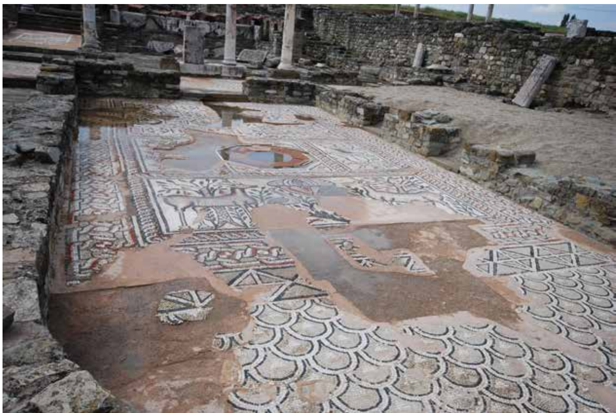
Fig. 49. Risks from atmospheric influences: degradation of the discovered buildings caused by rainwater
