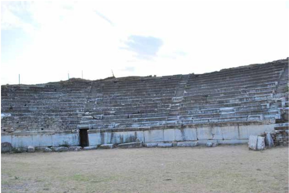
Fig. 52-53. Risk from air pollution: black surface on marble blocks at the Theatre caused by exhaust gases of the vehicles on the highway
