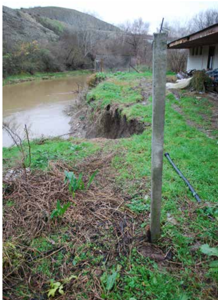
Fig. 38-39. Risk from flooding: collapse of the bank of Crna River adjacent to Depot 5, 2014
