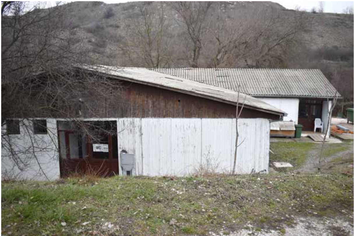
Fig. 100a. Storage facilities: depots 1, 3 and 4
