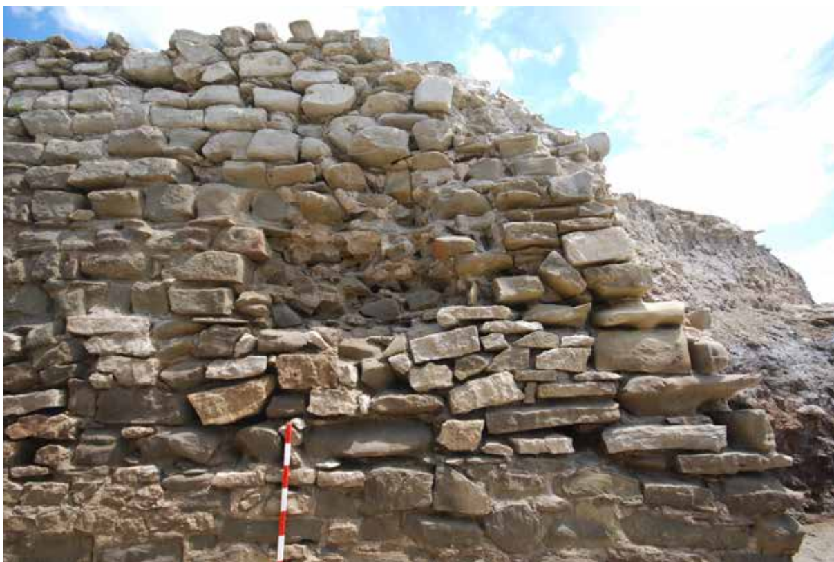
Fig. 50-51. Risks from atmospheric influences: poor quality building material – soft sandstone
