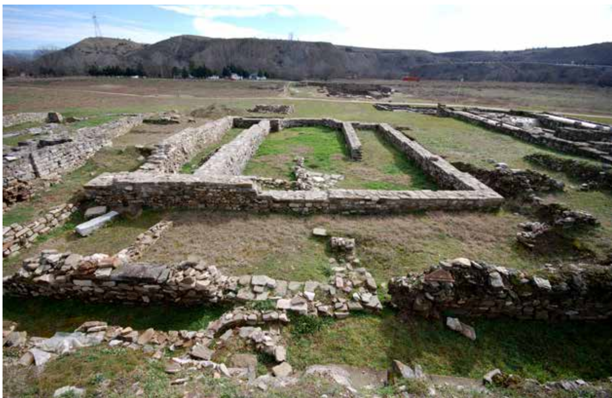
Fig. 92b. Civil Basilica, view from W
